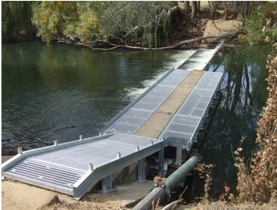
Figure 12. Irrigation weir ( www.pumpindustry.com.au/weir-upgrade-supports-irrigation )
