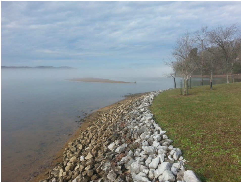
Figure 13. Hard armouring as riverbank protection ( https://trapbag.com/natural-materials-for-riverbank-protection )
