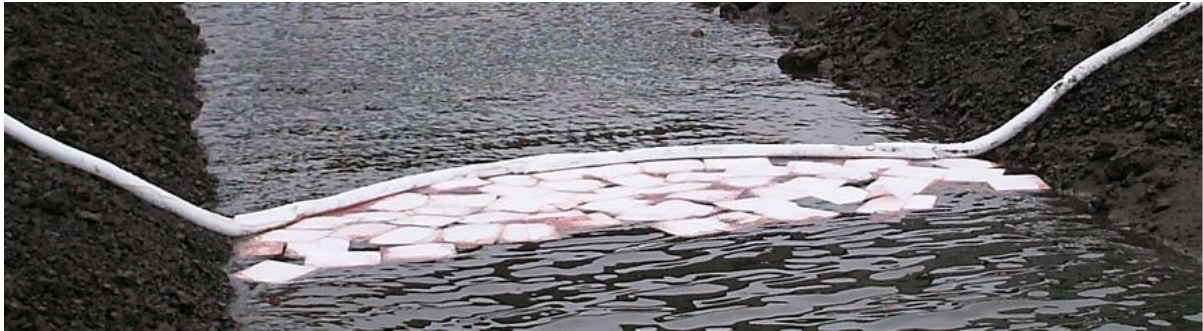
Figure 24. Use of sorbents for oil spill recovery ( https://foxdesignsg4fong.weebly.com/chemical-clean-up-methods.html )
