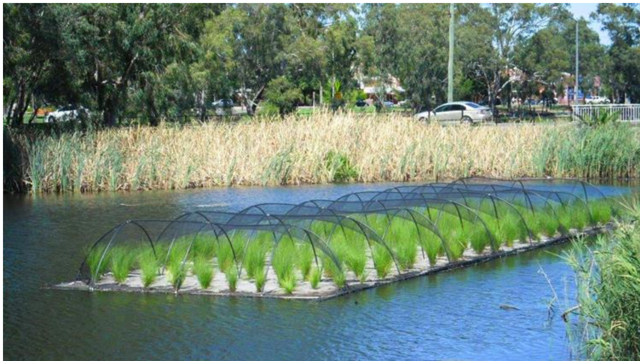
Figure 19. Ecological floating bed ( www.aquabiofilter.com )
